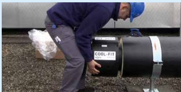
Slide-on the shrink sleeves and push the pipe ends up to the stop into the electrofusion coupler.
