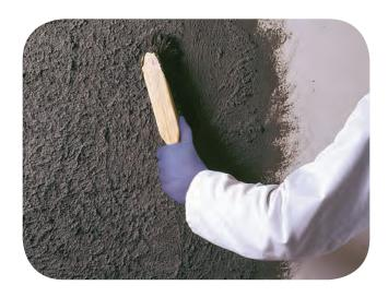
To avoid the risk of cracking, it is essential that certain considerations are taken into account prior to and during the application of render. This section, aimed at the monocouche applicator, focuses on good practice when preparing a substrate and applying the monocouche render.
