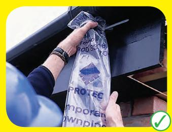
If one area of the wall is allowed to become soaked while the adjacent area is dry, the differential movement will cause stresses to increase and cracks to form.
