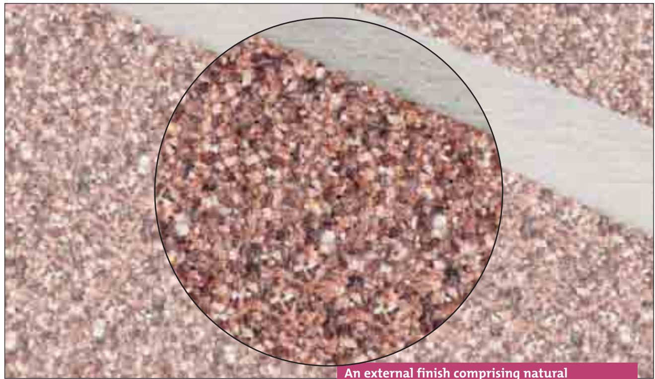
An external finish comprising natural aggregates bound in a clear resin binder
