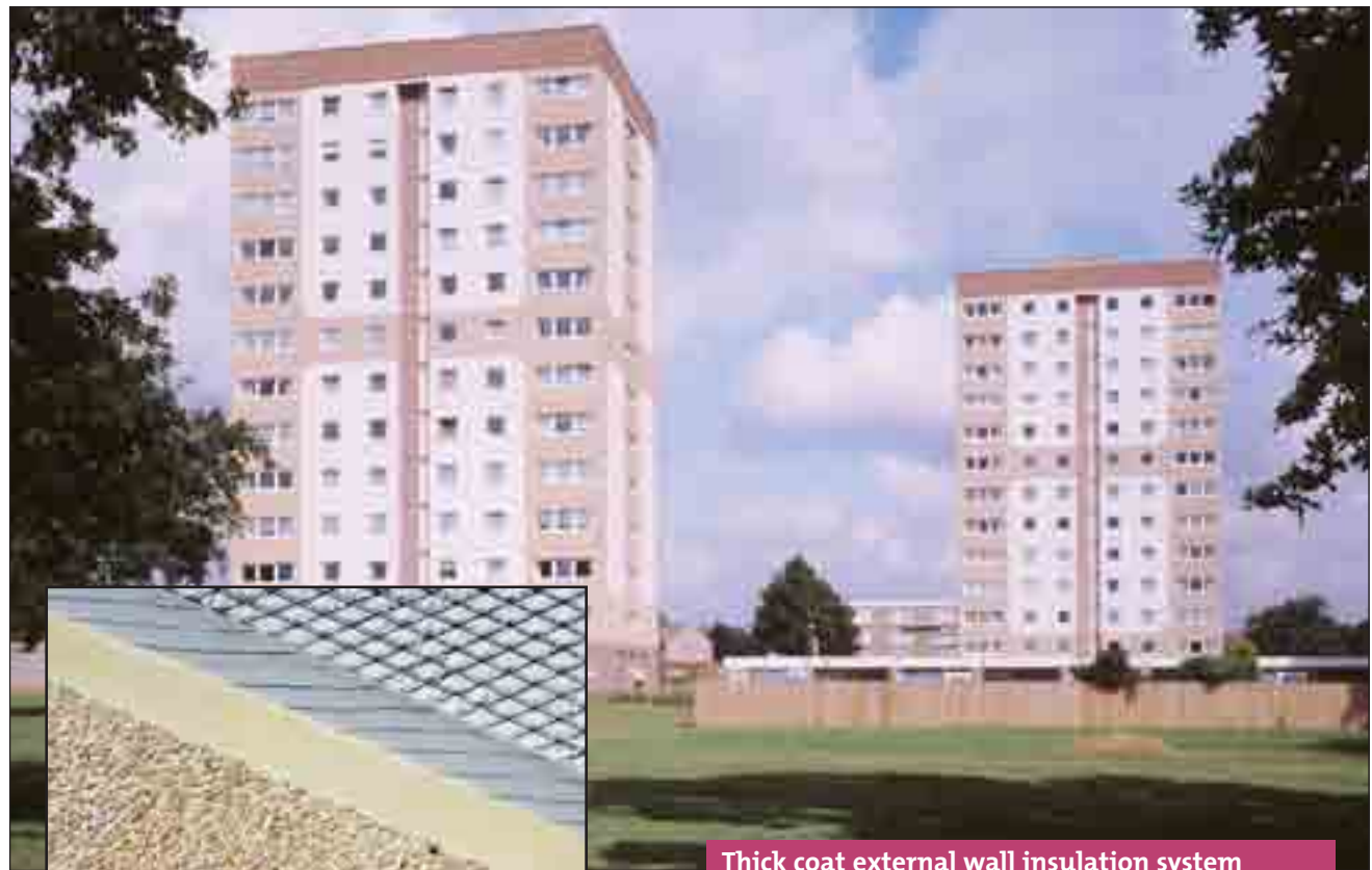
Thick coat external wall insulation system incorporating expanded metal lath
