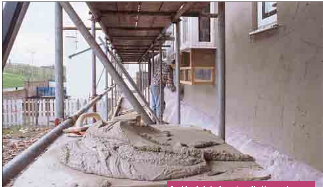
Pre-blended single coat application renders
