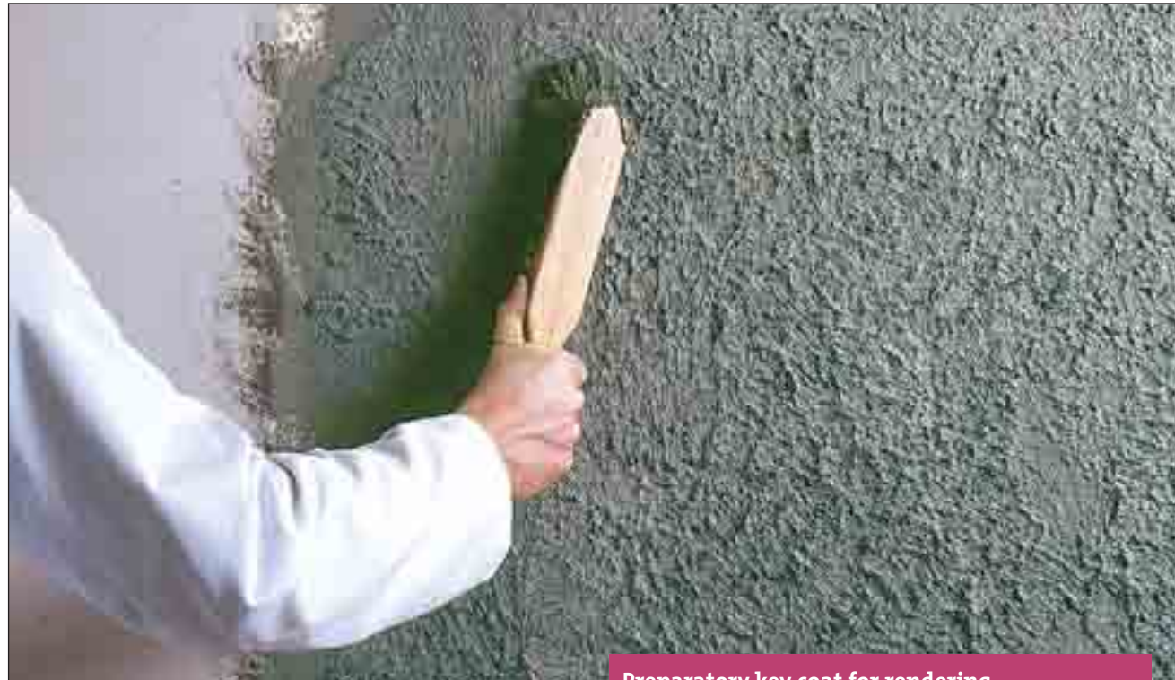
Preparatory key coat for rendering
