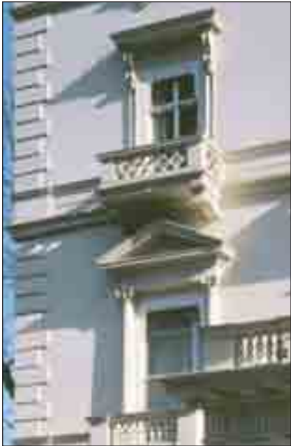
Project The French Embassy Location Portland Street, London Specifier The Heritage Division of Makers Industrial Client English Heritage System Applied direct to existing coatings, isolated re-profiling with renovex P. Finish santane EFL Features The removal of existing finishes proved impossible to carry out without damage to the underlying building fabric. santane's ability to be applied over all existing coatings, fine cracking and new re-profiling work saved the client considerable expenditure and disruption while completely satisfying English Heritage's requirement to avoid any material alteration to the facade.
