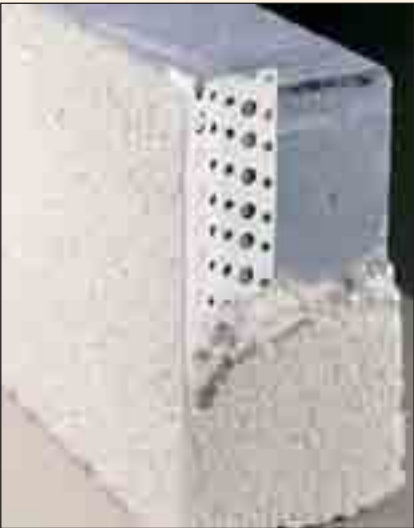
Y-section corner bead
