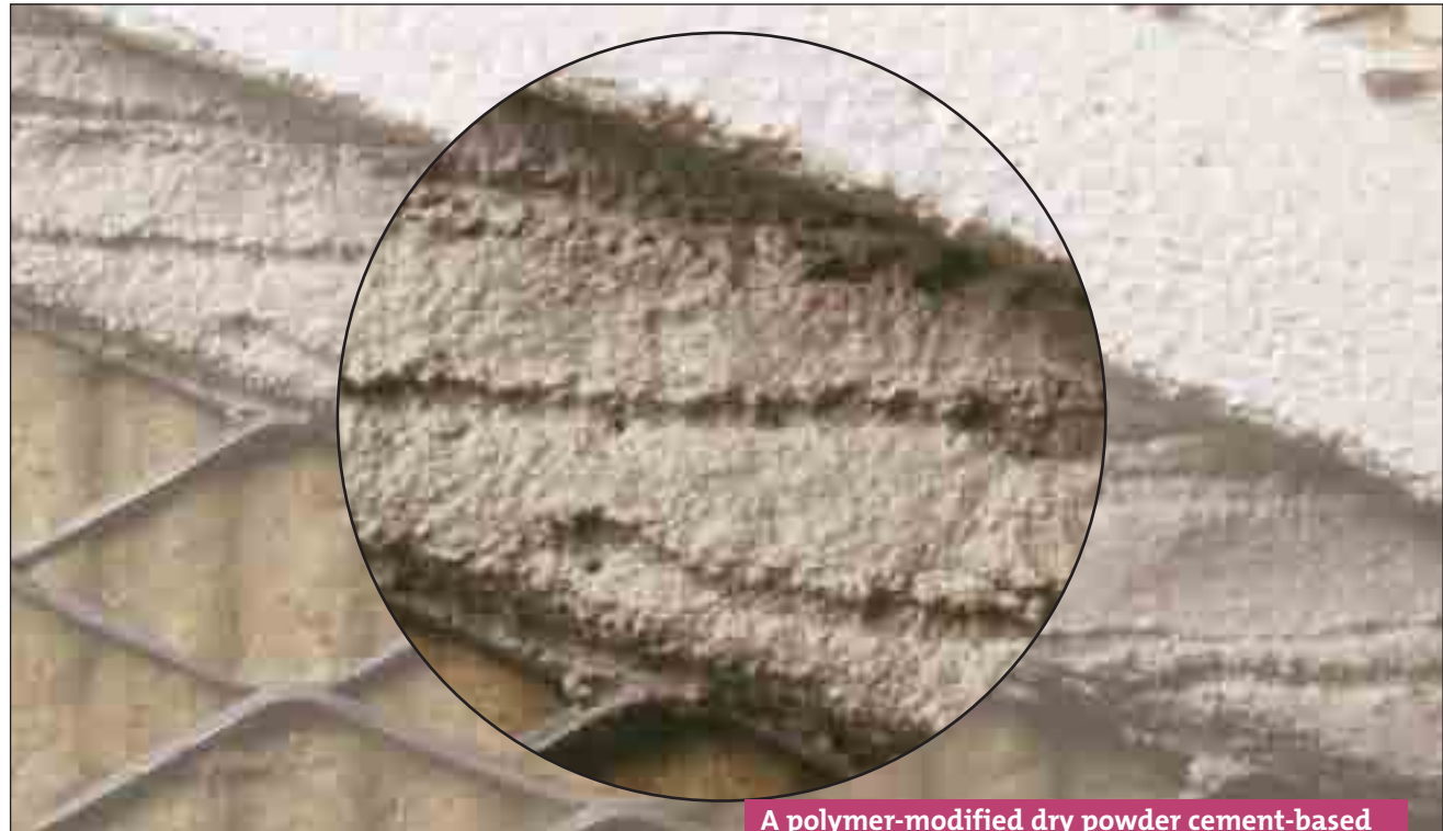
A polymer-modified dry powder cement-based mortar for use as a render undercoat on mineral fibre insulation
