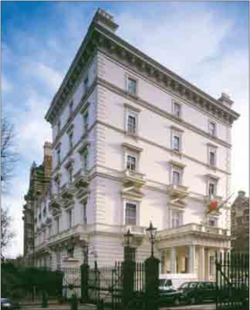
Project The French Embassy Location Portland Street, London Specifier The Heritage Division of Makers Industrial Client English Heritage System Applied direct to existing coatings, isolated re-profiling with renovex P. Finish santane EFL Features The removal of existing finishes proved impossible to carry out without damage to the underlying building fabric. santane's ability to be applied over all existing coatings, fine cracking and new re-profiling work saved the client considerable expenditure and disruption while completely satisfying English Heritage's requirement to avoid any material alteration to the facade.
