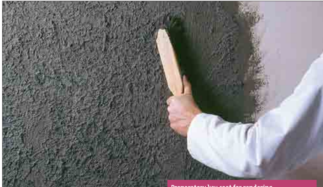
Preparatory key coat for rendering
