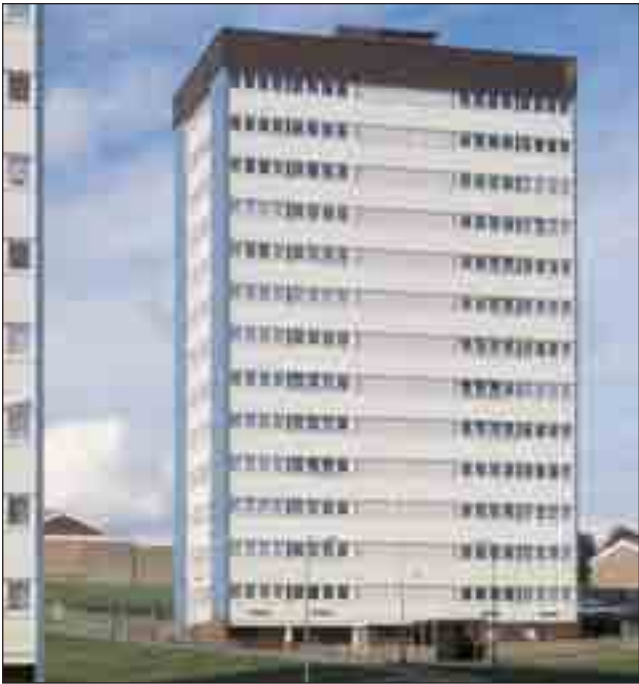
Project Giles Close House Location Birmingham Client Birmingham City Council System Applied direct to mosaics levelling where necessary with renovex P Finish santane Features One of three in the same development and just a sample of others treated for the Council, existing mosaics were secured and the properties refurbished incorporating meshcloth in the santane system. Selective use of bold colour dramatically improves the visual impact of the typical Local Authority high-density, multi-storey accommodation.
