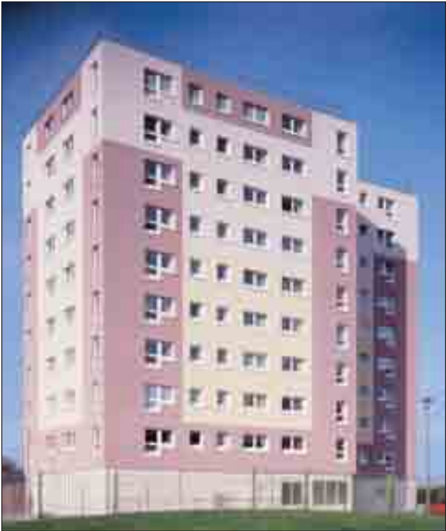
Project Jupiter, Milford and Portland Courts Location Middlesbrough Specifier Middlesbrough Council System weber.therm XM Finish weber.sil TF 1.5 mm Features Following extensive repair of the concrete fabric of the tower block, the building was refurbished without disruption to the residents, stabilising the structure and bringing insulation standards nearer to current requirements.
