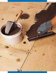
Grouting a plywood substrate with Nivorapid + Latex Plus
