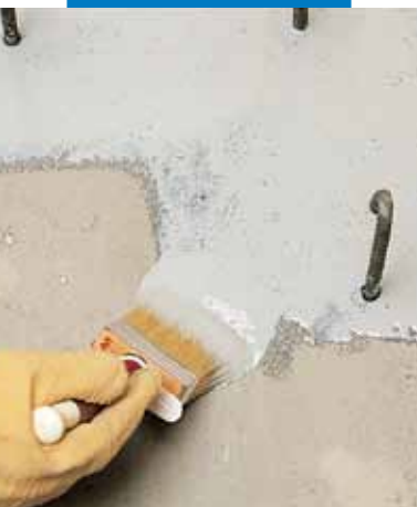
Applying Eporip by brush on construction joint
