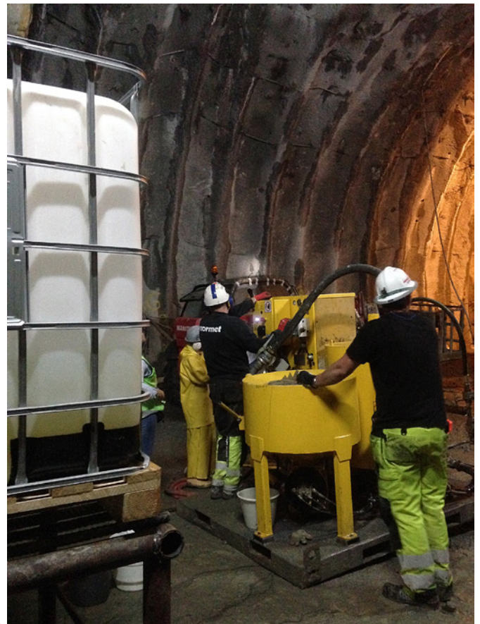
TamCrete 400CS secondary grouting
