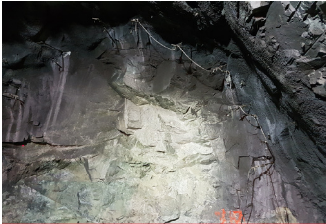
TamCrete MFC pre-excavation grouting using chained off packers
