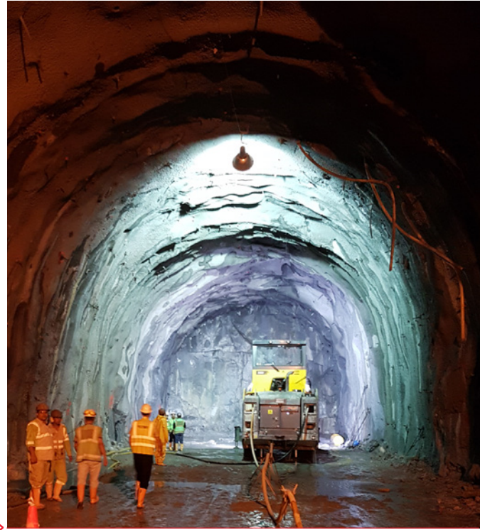
Pre-injection grouting with TamCrete MFC
