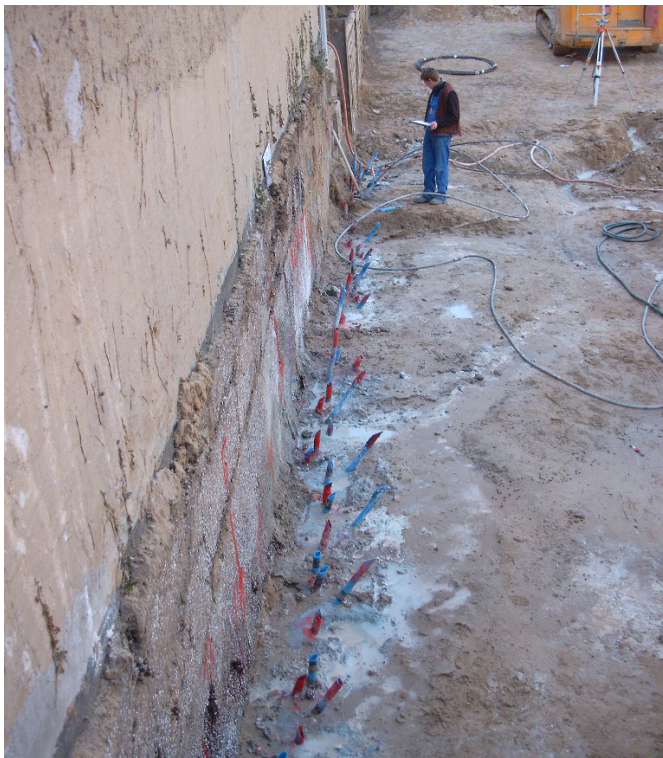
Foundation grouting with TamCrete UFC
