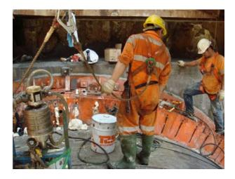
TamPur 130 / TamKat 130 is a single-shot hydrophobic polyurethane based on MDI in combination with polyether polyols and an amine based catalyst. The system only reacts when it comes into contact with water, producing a non-toxic, semi-flexible polyurethane foam.
