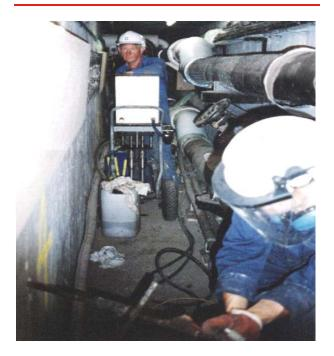
TamAcryl 2000 is a blend of acrylic polymers used in conjunction with an accelerator and catalyst system. Upon mixing of the components, a chemical reaction occurs and a waterproof gel is formed. It is available in two grades standard and slow set.
