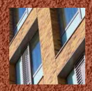
Designed to create a lightweight, natural brick appearance, Gebrik insulates and protects a building from water penetration and is siteapplied to buildings constructed of masonry, timber, steel frame or SIPs to clad new buildings or refurbish and protect existing buildings.
