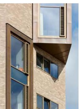
structural support required over the building from around 200kg/m² of brickwork to around 50kg/m² of Gebrik. In addition to lower scaffold and structural support costs, Gebrik also contributed to a reduction in prelim costs, thanks to its impressive speed of installation.
