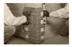
A corner piece is typically the first element to be installed which, when combined with the starter rail, sets a right angle for installation of the first row of elements.
