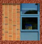
Gebrik's insulating properties will help to significantly improve a building's thermal performance (it is proven to reduce a building's U-value by up to 60%) and keep wall thickness to a minimum. The insulating material is polyurethane (PUR) and uses pentane as its blowing agent and therefore does not release CFC or **HCFC** agents during manufacture. The PUR has a BREEAM element number of 815320017 and Green Guide rating of A.
