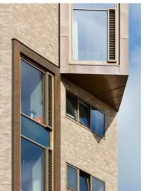
structural support required over the building from around 200kg/m² of brickwork to around 50kg/m² of Gebrik. In addition to lower scaffold and structural support costs, Gebrik also contributed to a reduction in prelim costs, thanks to its impressive speed of installation.
