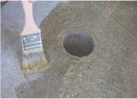
2- Prime the whole surface area of the substrate according to the waterproofing system specifications.
