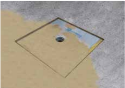
6- Apply the Alsan® waterproofing system as far as the opening.
