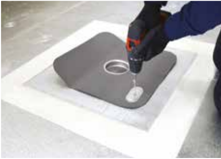
3- Mechanically attach the Draini® Flag flange. One fastening on each corner.
