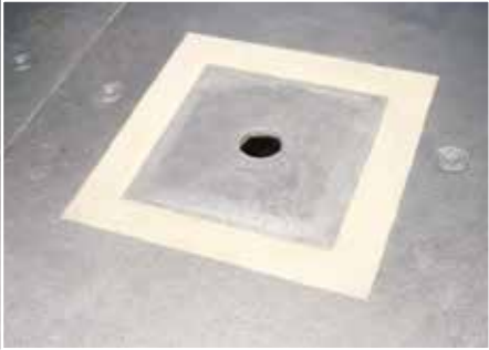
1- Cut out an area in the insulation.
