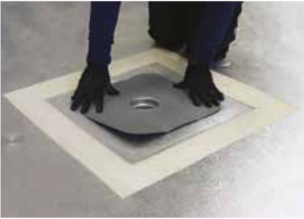
2- Insert Draini® Flag into the drain pipe after laying the waterproofing layer, only for felted membranes.
