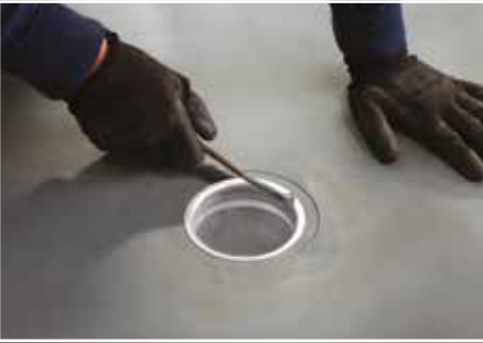
4- Check the welding using a Flag Welding Tester .
