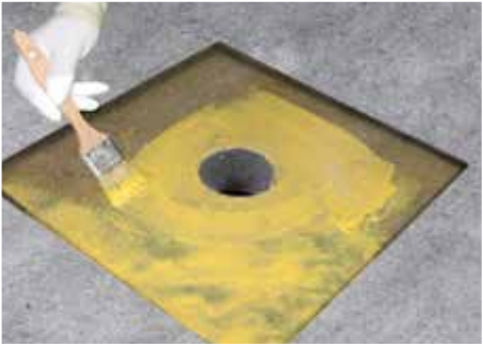
3- Once dry, apply a layer of Alsan PMMA or PU primer for the surface. Then Alsan PMMA 770TX or Alsan 601 PU coating
