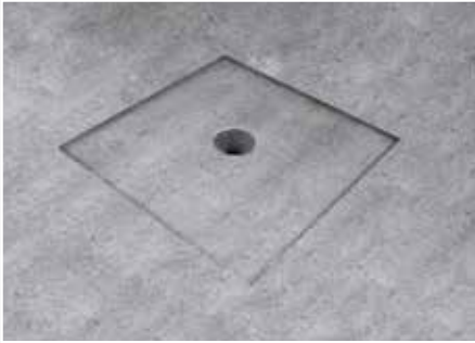
1- Cut out an area 35 cm x 35 cm, then cut a chamfered edge at the outlet point.
