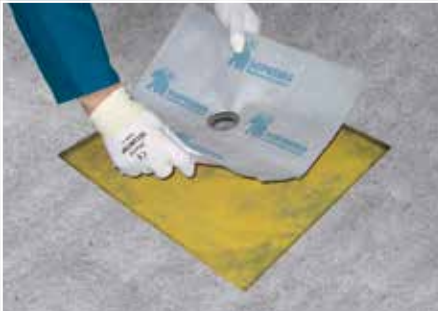
4- Insert the Draini Alsan® pipe into its groove.
