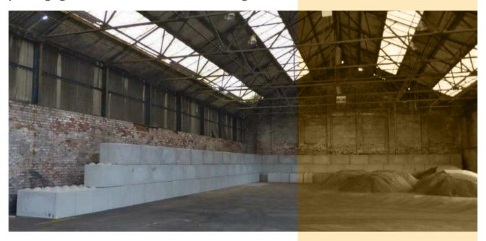
The building would have to be demolished but there was a requirement for something to strengthen the inner part of the building whilst keeping a proportion of the existing brickwork to a set height - then the roof and metalwork could be safely taken down.
