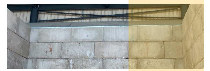
One of RSG's clients required the construction of a high walled (6 or 7m high), covered bunker. The site of the new bunker already had a solid slab base. However the existing slab had many different levels meaning putting walls directly on it would be an issue.
