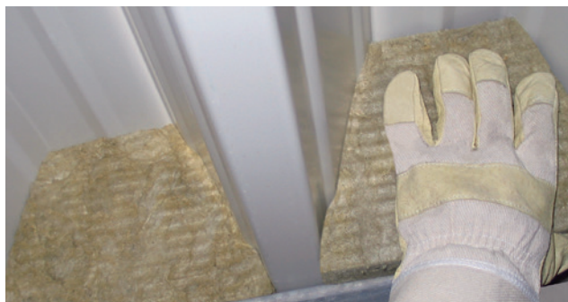
Installation example: ISO-PROFIL FILLER PIECES
