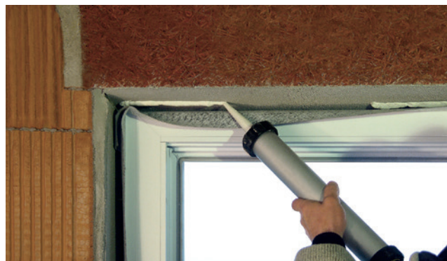
Installation example: ISO-TOP FLEX-ADHESIVE SP
