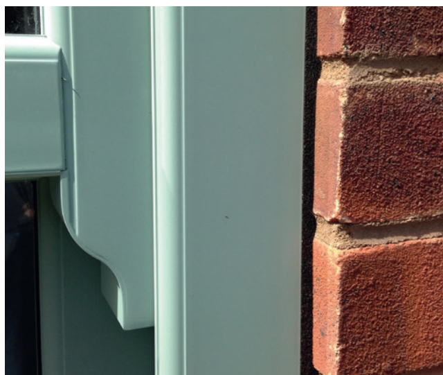
Installation example: ISO-BLOCO WIN2WALL
