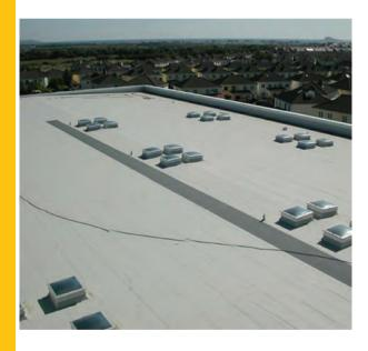
Comprising a range of single ply membranes that can be attached in a number of ways, the **Sika-Trocal** Concept is suitable for most forms of flat, pitched, curved or even vertical roof surfaces.
