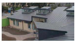
The **Sika-Trocal** adhered system uses **Type SGK** membrane, which has an integral polyester fleece backing that helps mask the appearance of insulation board or timber deck joints. The **Type SGK** membrane is adhered to the substrate using **Sika-Trocal Type C300** polyurethane adhesive.
