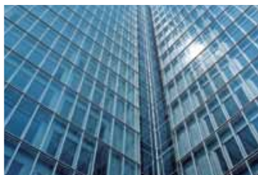
Sealing of glass façades
