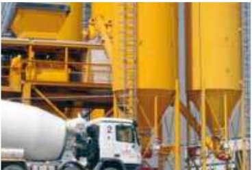
Ready-mix concrete production
