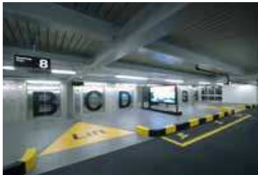
Flooring in car park decks
