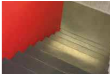
Flooring for vomitories and stairways
