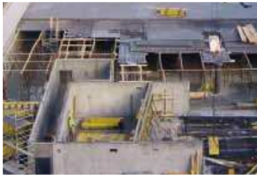
Watertight concrete for basement waterproofing
