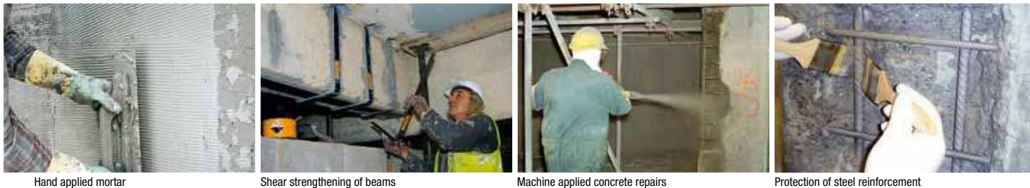
Hand applied mortar
