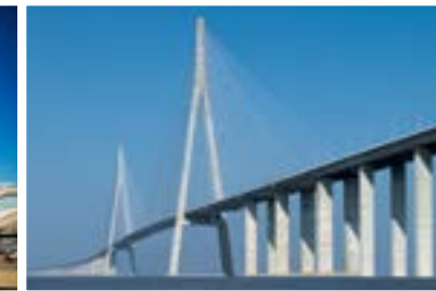
Suton Bridge, China
