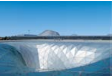
Weather sealing of glass and metal cladding
