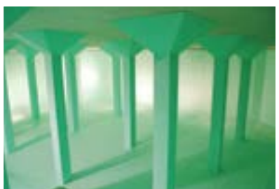
Waterproofing for drinking water facilities
