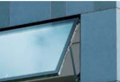
Structural window bonding
