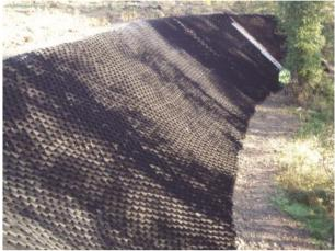
The Verdacell may be laid in either direction. Stretch the Verdacell down the face of the slope and pin in position according to the specified pinning pattern. One fixing pin to each cell in top trench. One fixing pin to every other cell at bottom. Should the slope be more than 2.5 m long intermediate fixing ties or pins may be required.
