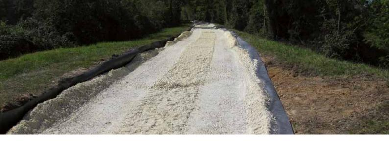
DuPont™ Plantex® RootProtector is a water-permeable root barrier.
